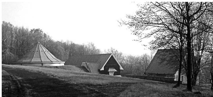
**Figure 9** The geomagnetic observatory of Dourbes, showing the construction of the pavilions housing the observing instruments. To the left is the underground vault for the variometers: a high thermal inertia coupled with thick insulation ensures a low daily temperature variation in the vault. In the center is the absolute measurement pavilion, housing the reference pillar for the observatory. To the right, a technical pavilion for mains appliances and offices.
